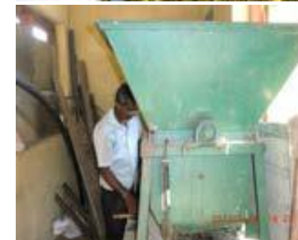
Figure 3: The digester feeding point
