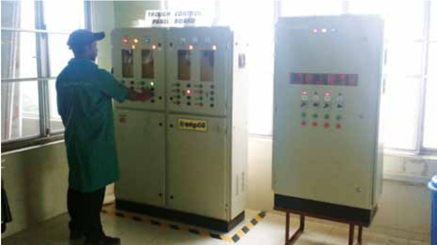
Figure 4: VSD Controlled withering troughs
